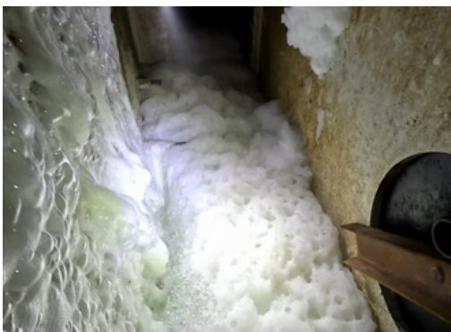
Chemistry reacting in a unit
